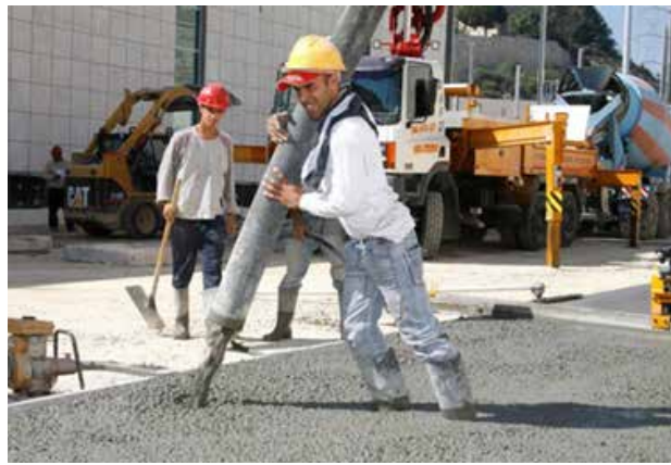
Sand is a key ingredient in the making of concrete
