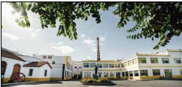
'Kendel receive further MAJOR Order from Arehucas Rum factory on Gran Canaria.'
