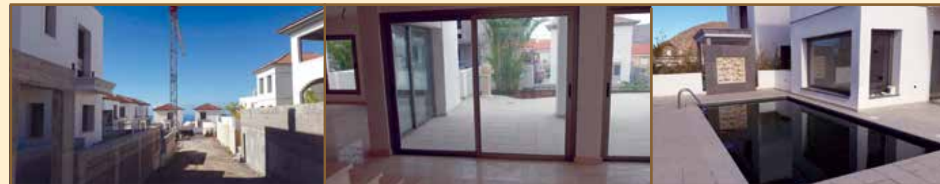
Photographs: Complex under construction, lounge and patio near completion and swimming pool.
