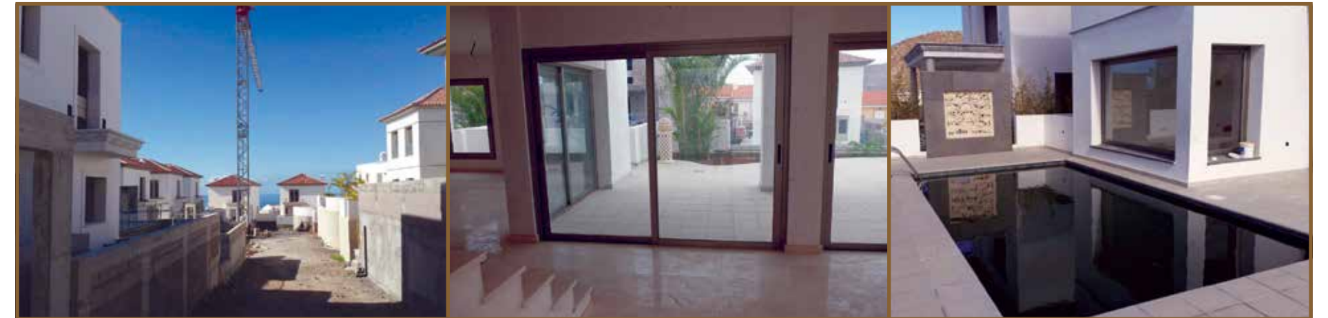
Photographs: Complex under construction, lounge and patio near completion and swimming pool.
