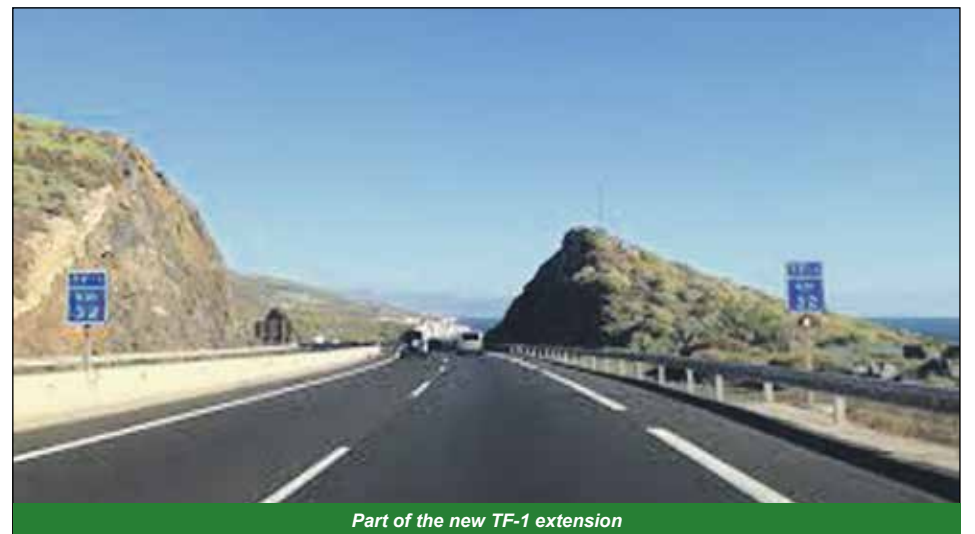
Part of the new TF-1 extension
