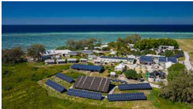
The island's solar power station generates enough renewable energy to run the entire resort
